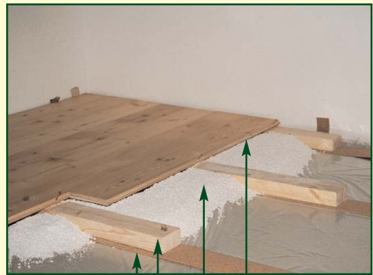
Felt or cork stripe Headless screw Floor timbers packing material
