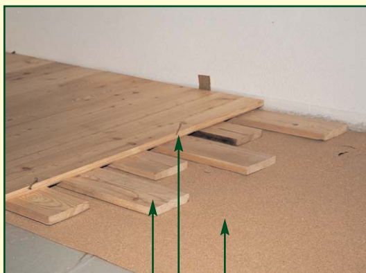
Smooth edged board Headless screw Felt or cork stripe
